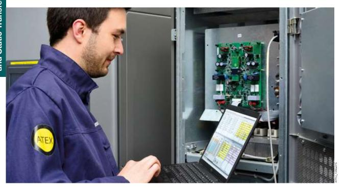
The commissioning of an STS covers start-up of the equipment, verification of its functions according to its design specifications, and to ensure that it is compatible with the customer's working environment.
