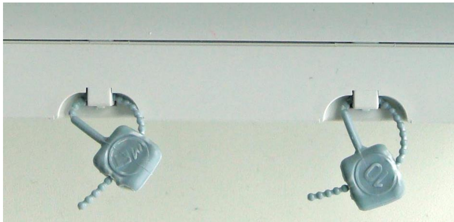
Figure 4 - Meter protection after installation
