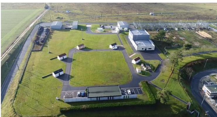
EDF's Concept Grid Network reproduced the installation of the Lérins Islands on a ¼ scale
