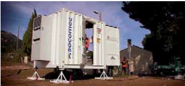
Easy to use, this 33-kW storage container is installed on the low-voltage network.
